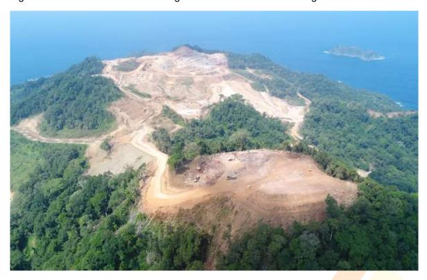
Figure 4 – Aerial view of Pit C and haul road access clearing and grubbing
