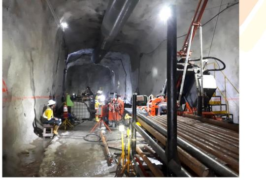
Drilling for hydrological investigation (MBH-20-041) purposes near the western edge of the Tujuh Bukit Copper Resource (Figure 3) encountered several well mineralised sections that may extend the current resource to the west.
