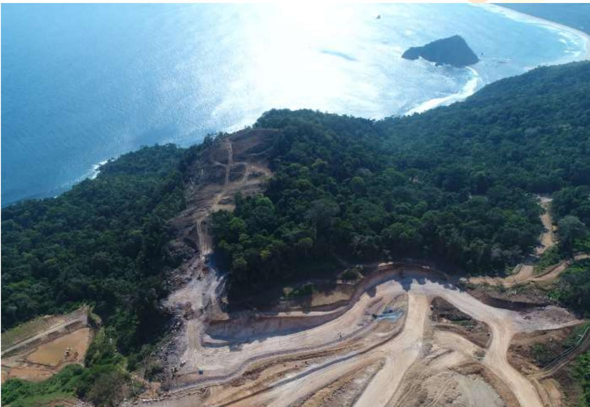
Figure 5 – Aerial view of the Heap Leach Pad showing Lift 3 nearing completion
