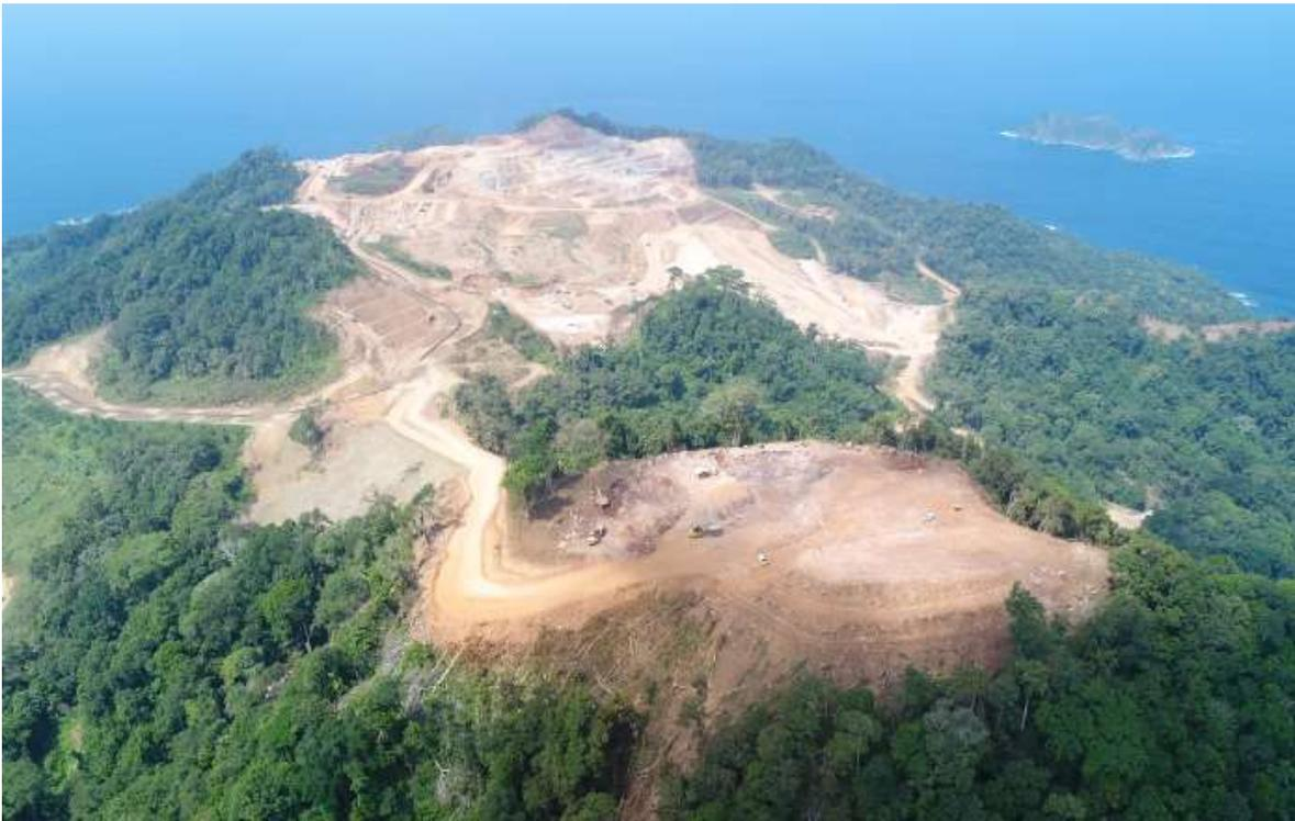
Figure 4 – Aerial view of Pit C and haul road access clearing and grubbing
