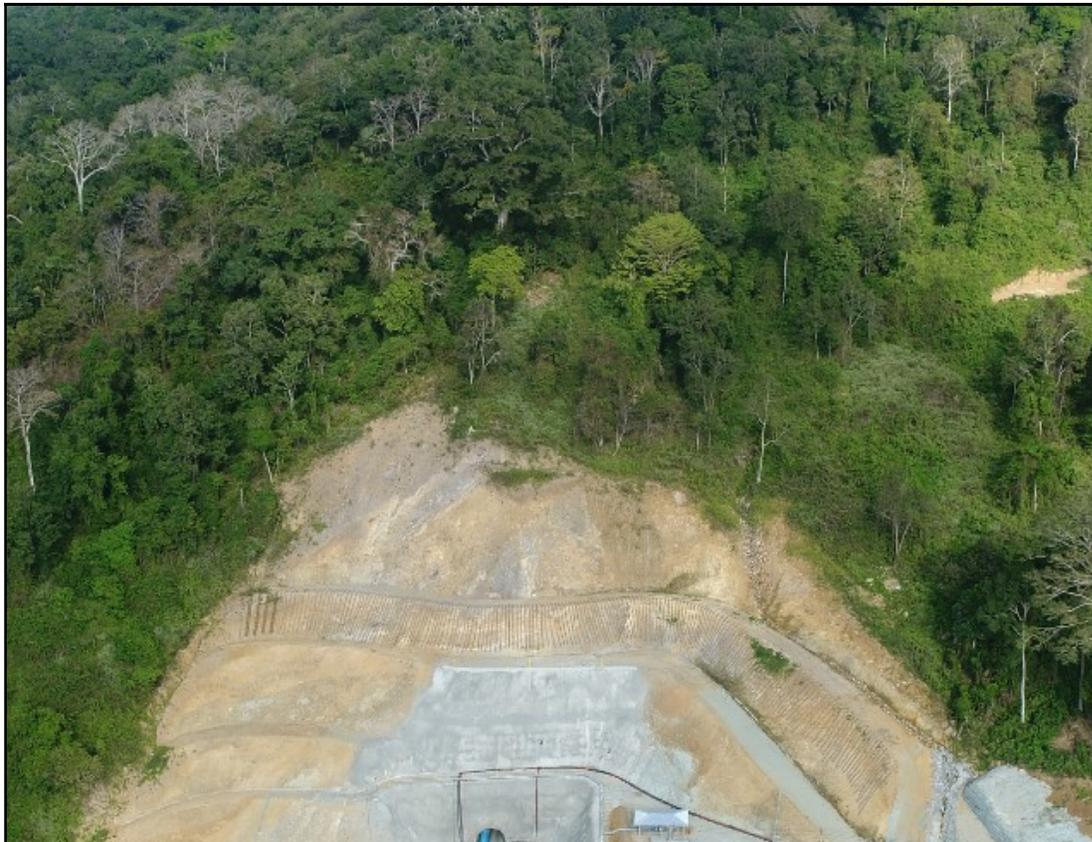
Figure 7 – OPP-2 bulk earthworks, slope stabilization and completion of the new workshop
