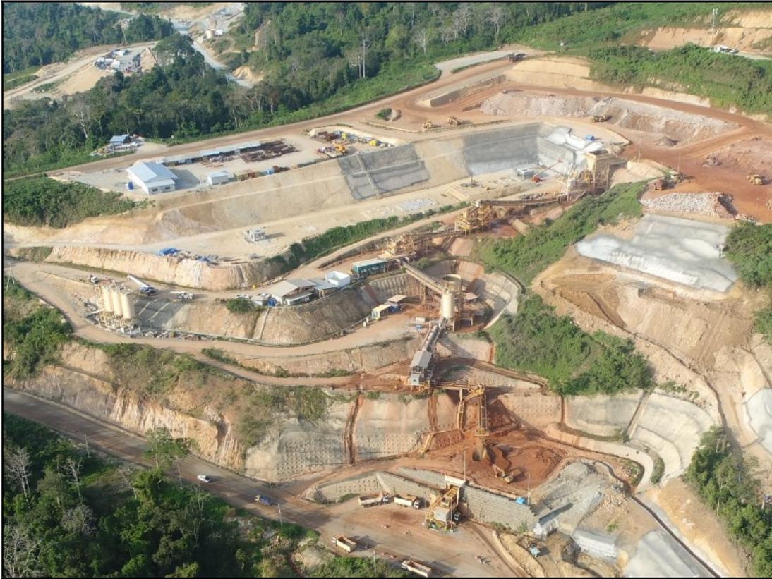
Figure 8 – HLP Stage 1B & 2B nearing completion, final placement of LLDPE liner at Stage 2B
