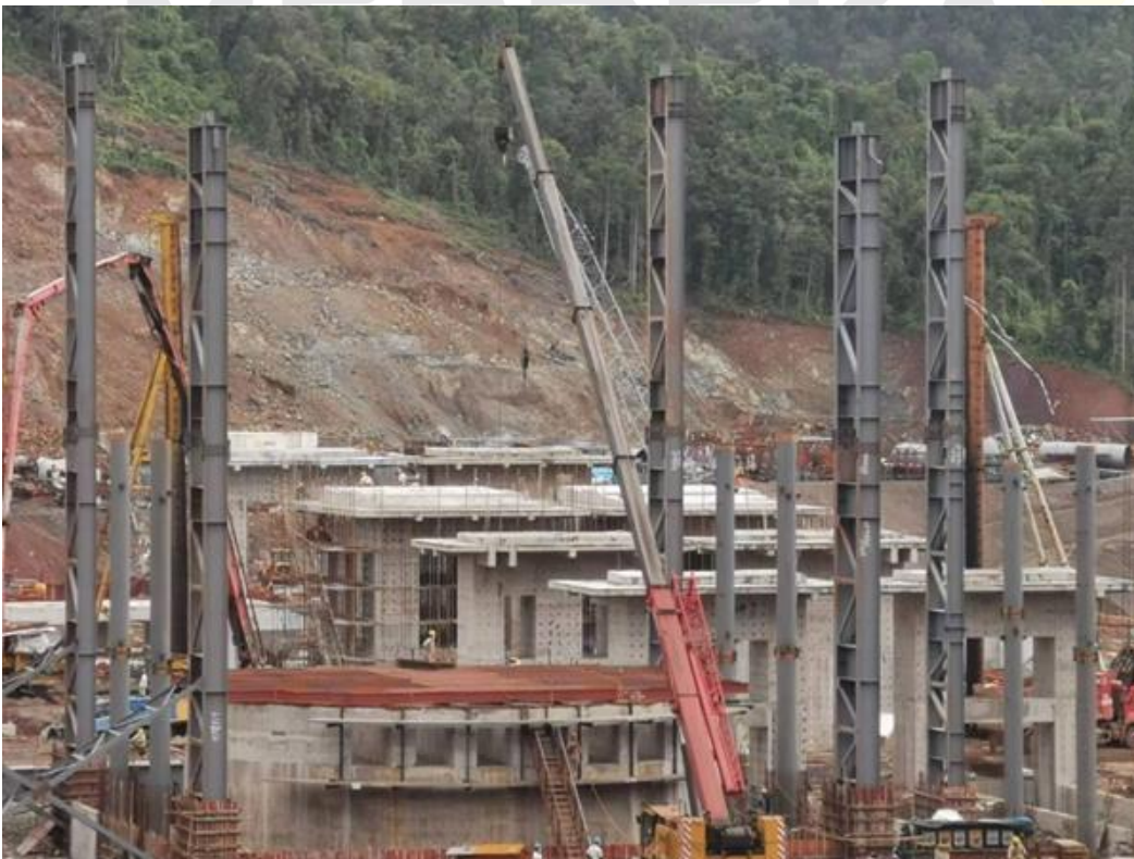
Figure 6: ZHNS RKEF construction progress
