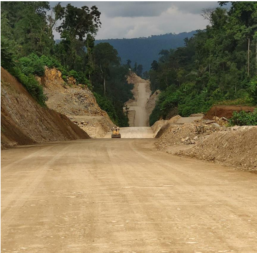
Figure 4: Physical progress of haul road
