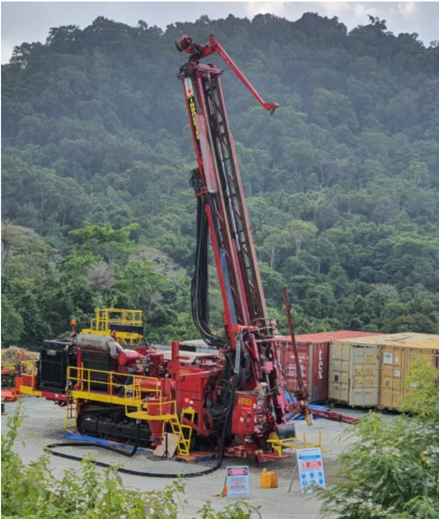
Figure 9: Additional RC rig undergoing site commissioning at Tujuh Bukit.
