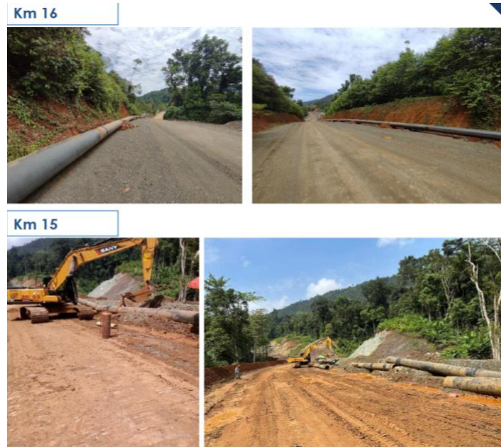
Figure 5: Slurry pipe installation
