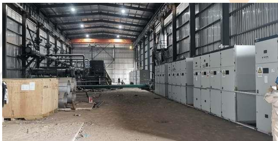
Figure 8: ZHN RKEF construction progress – air compressor room
