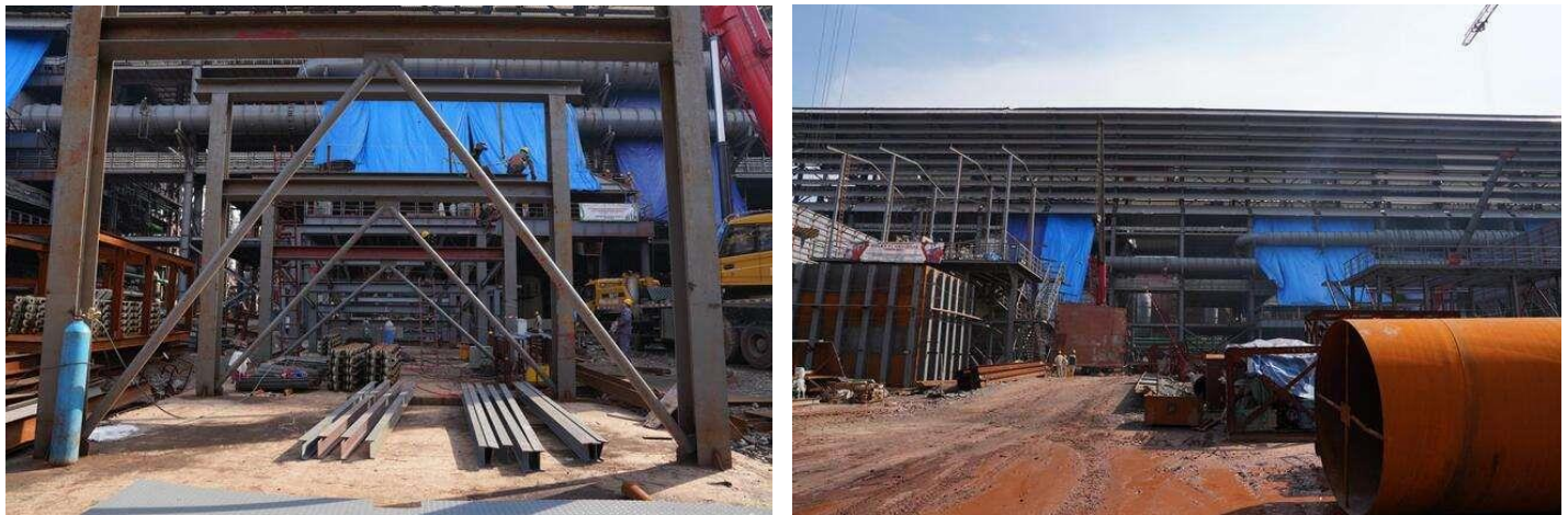
Figure 7: ZHN RKEF construction progress - Plant
