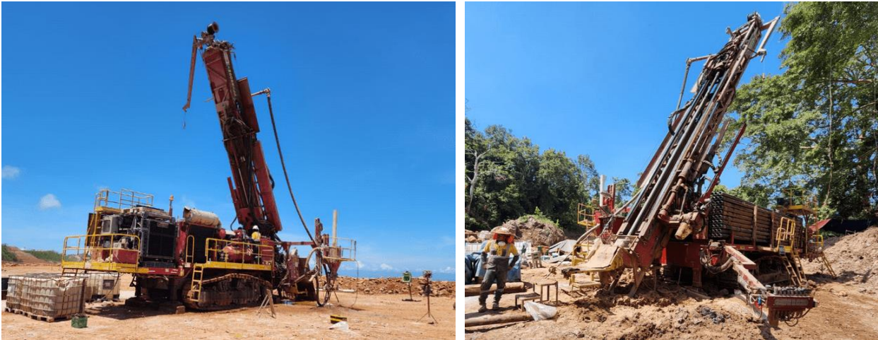
Figure 13: RC drilling into the Pit A highwall and along strike of Pit A
