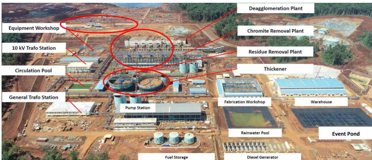
Figure 4: FPP Construction
