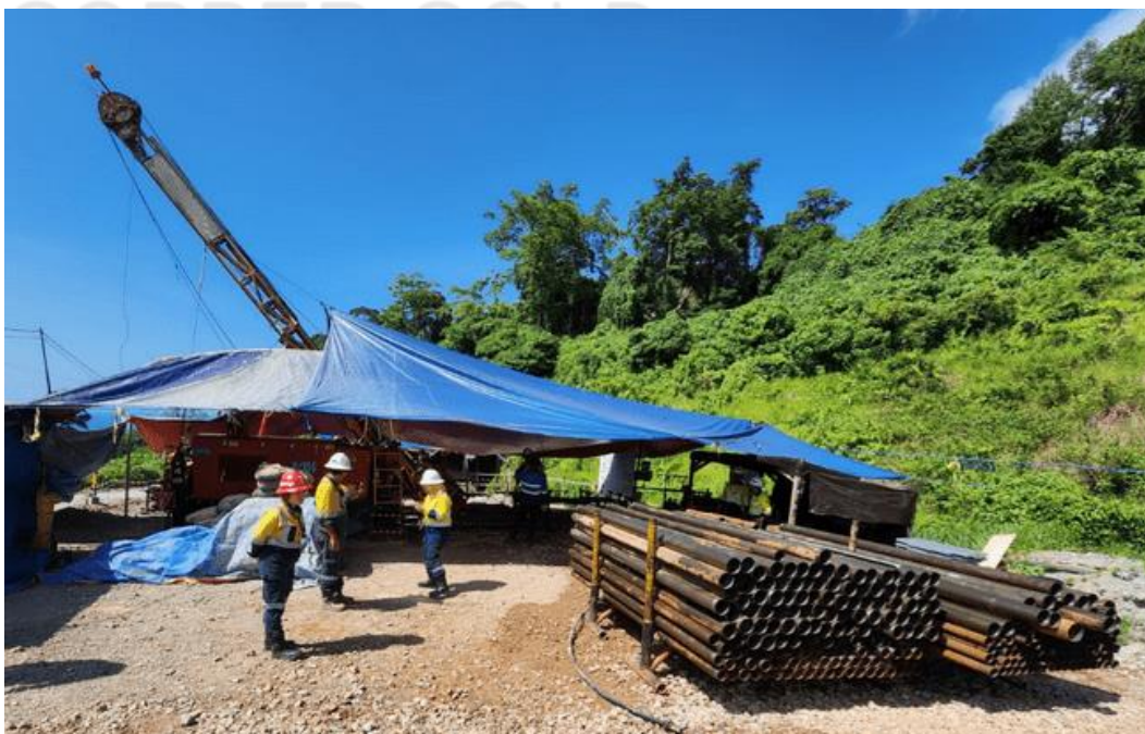
Figure 2: Surface drilling operations at Tujuh Bukit Copper Project
