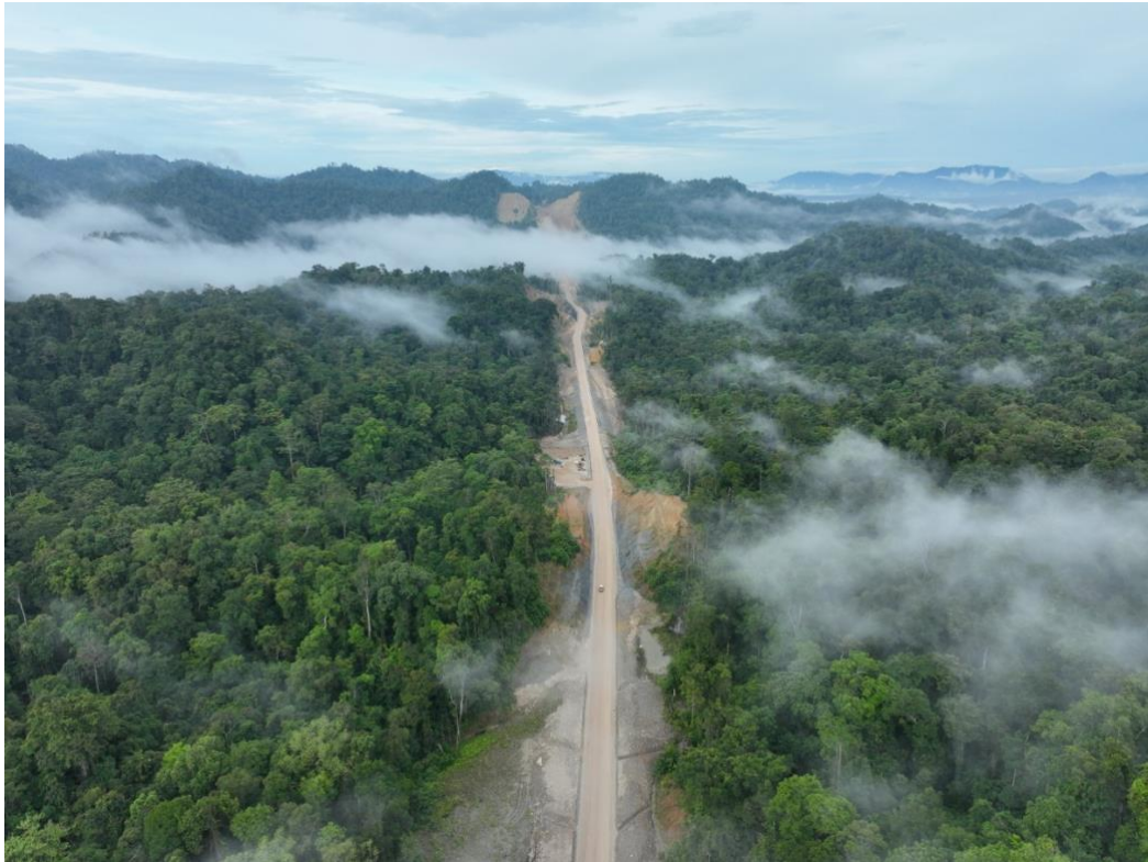
Figure 3: SCM haul road
