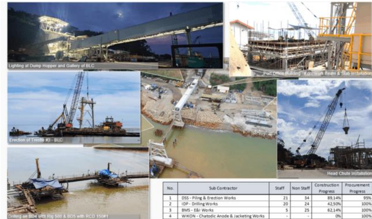
Figure 15: Wetar Barge Jetty
