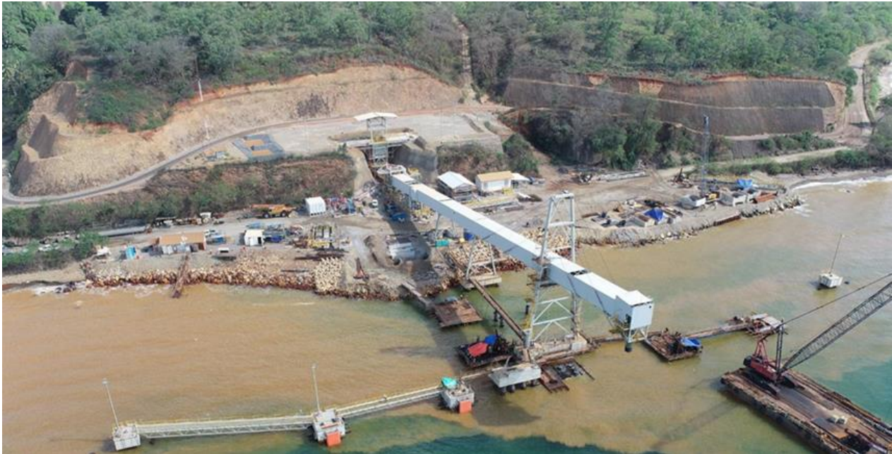
Figure 10: Wetar Barge Jetty
