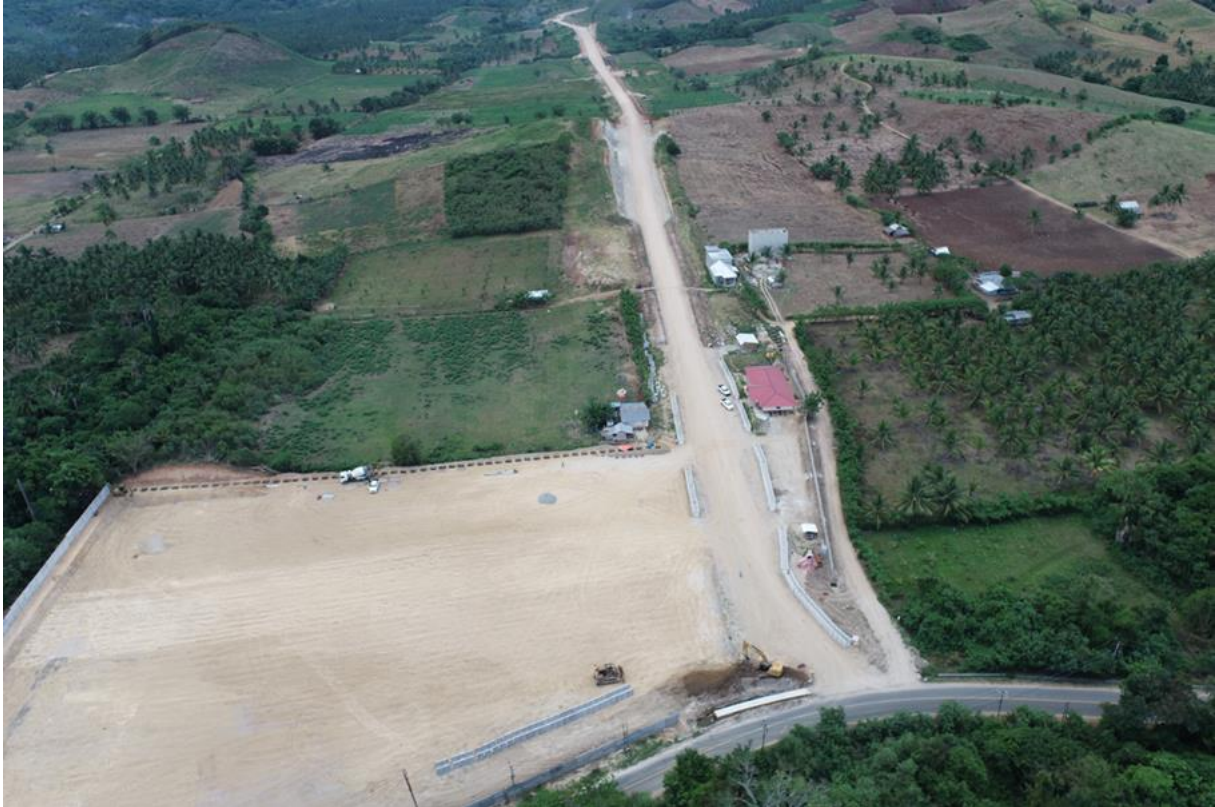
Figure 7: Bypass Road, connection to Trans Sulawesi Highway (11km to Mine Entrance)
