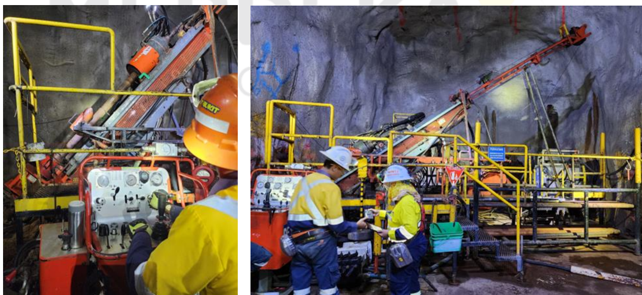
Figure 1: Underground drilling operations at Tujuh Bukit Copper Project
