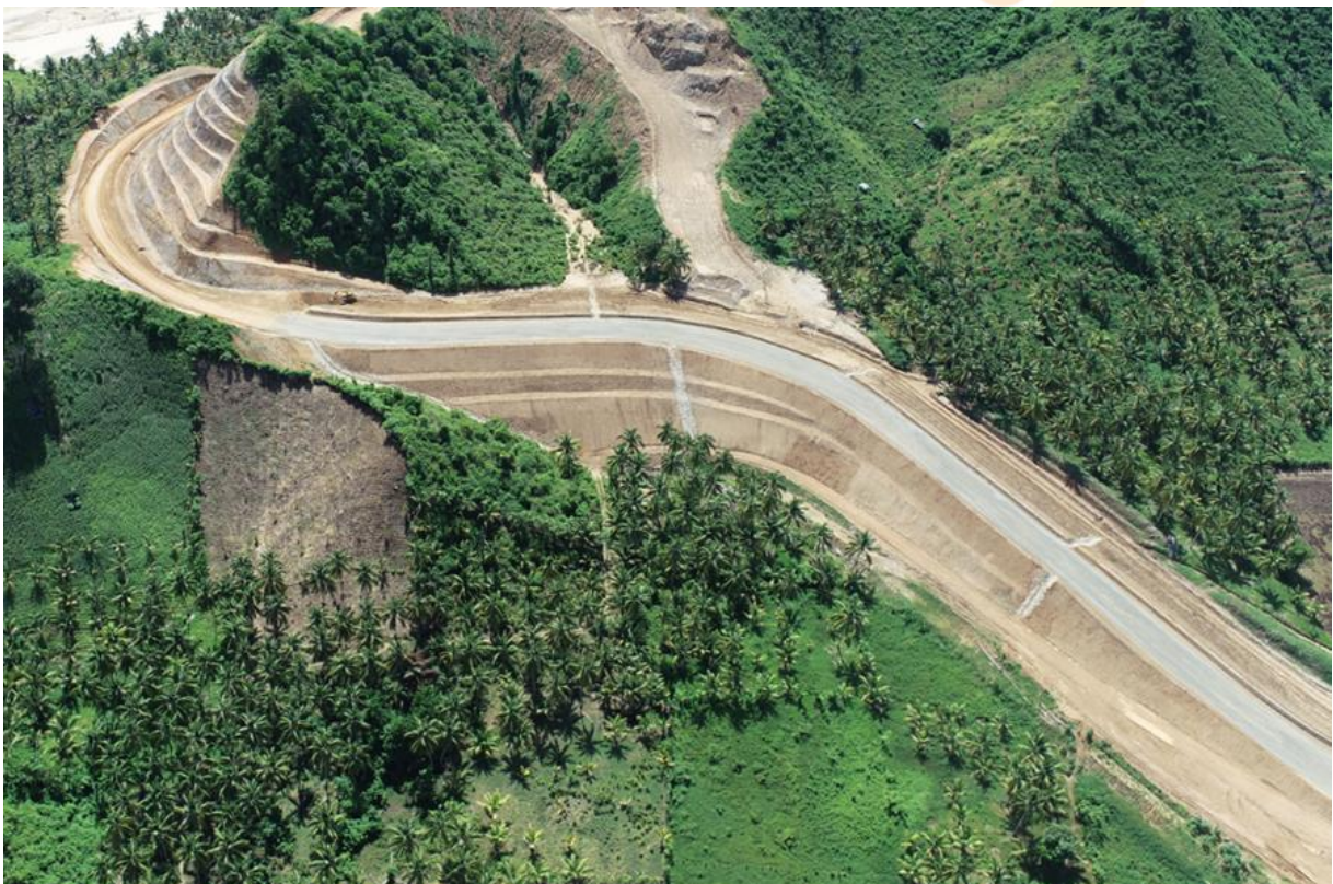
Figure 6: Bypass Road, approach to Mine Entrance
