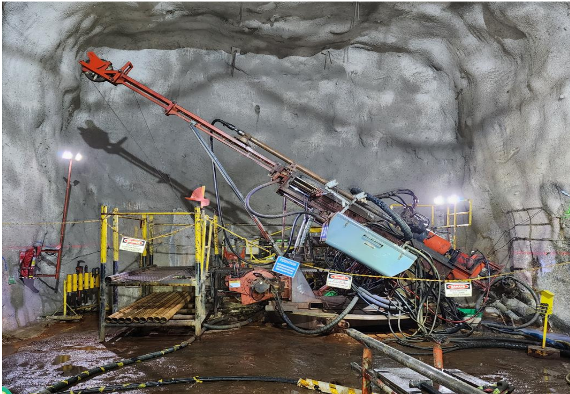
Figure 5: Resource definition drilling from underground
