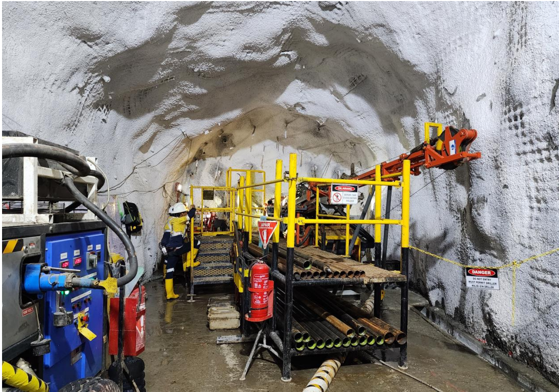
Figure 6: Drilling a decline cover hole to geotechnically assess ground conditions
