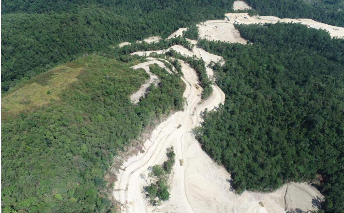
Figure 3: Pani main haul road construction
