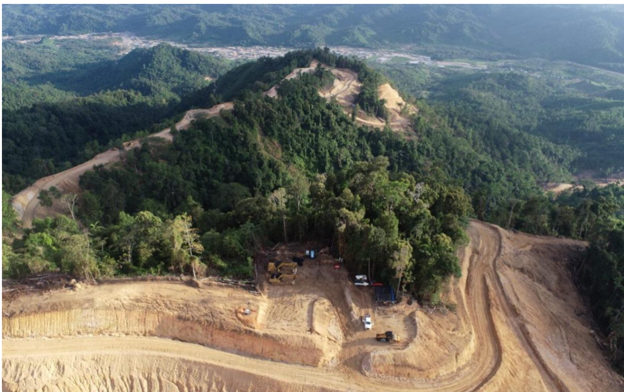
Figure 1: Mine hauling road construction
