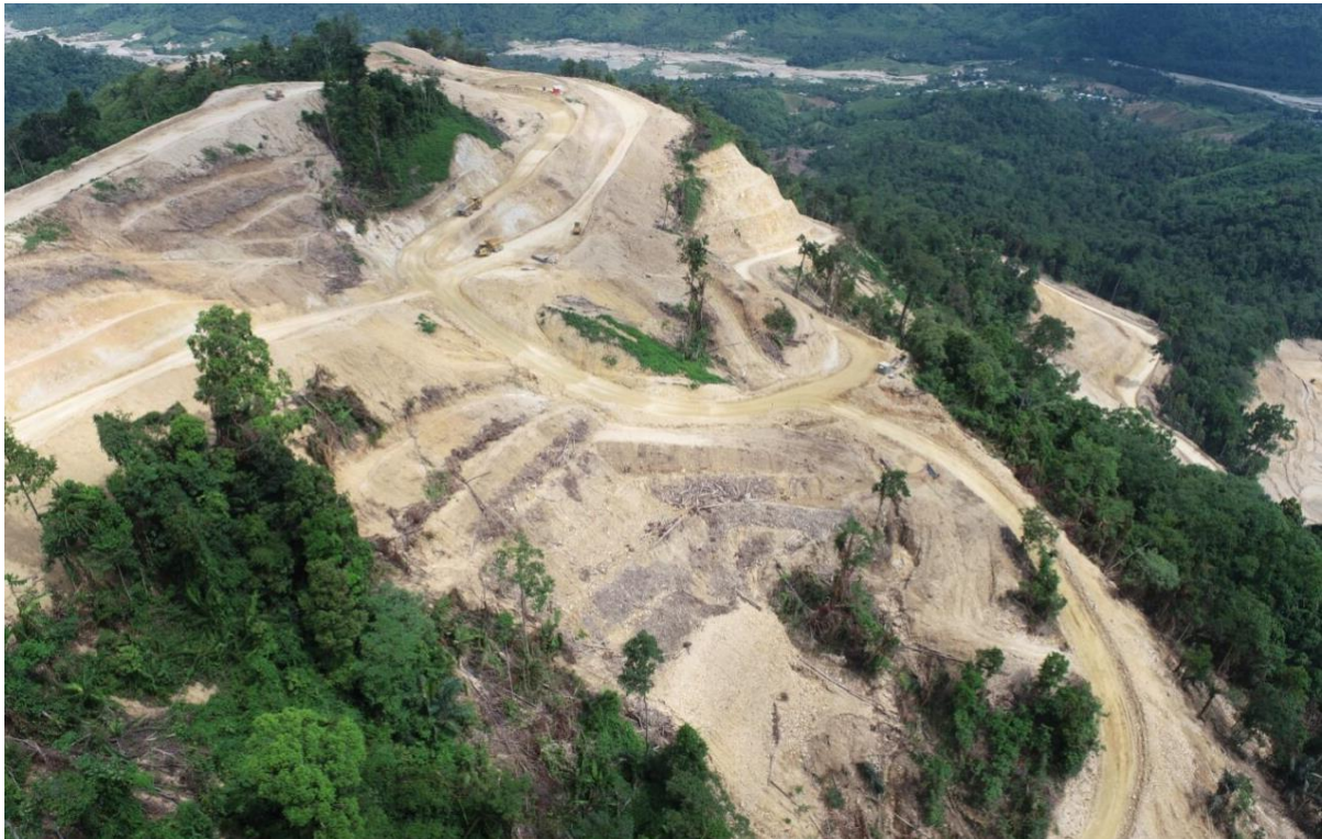
Figure 2: Mine hauling road construction
