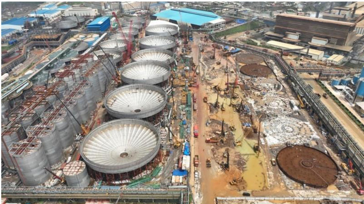
Figure 7: PT ESG HPAL plant construction progress
