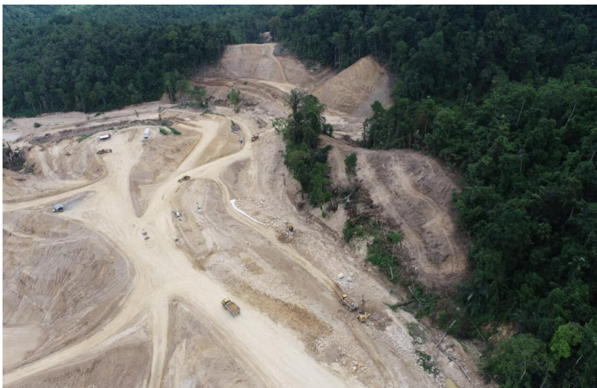
Figure 1: Ore processing plant construction
