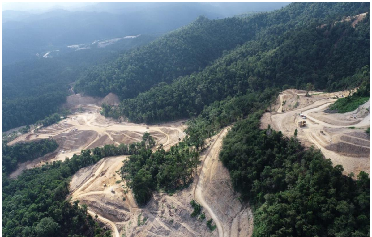
Figure 3: Ore processing plant and mine hauling road construction
