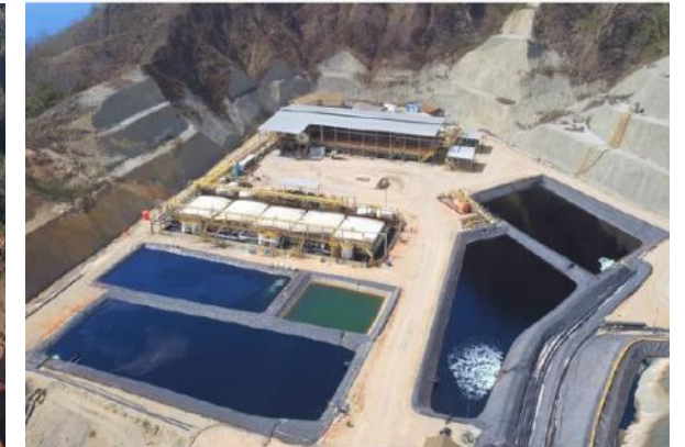
SX/EW Processing Plant
