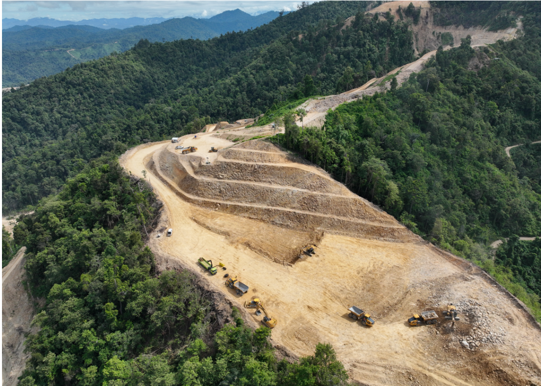
Figure 2: Mine hauling road construction
