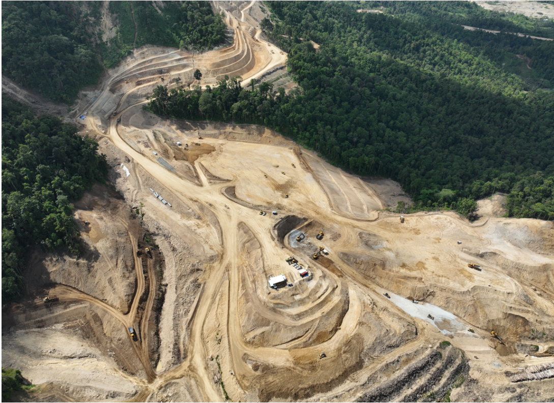
Figure 1: Ore processing plant construction
