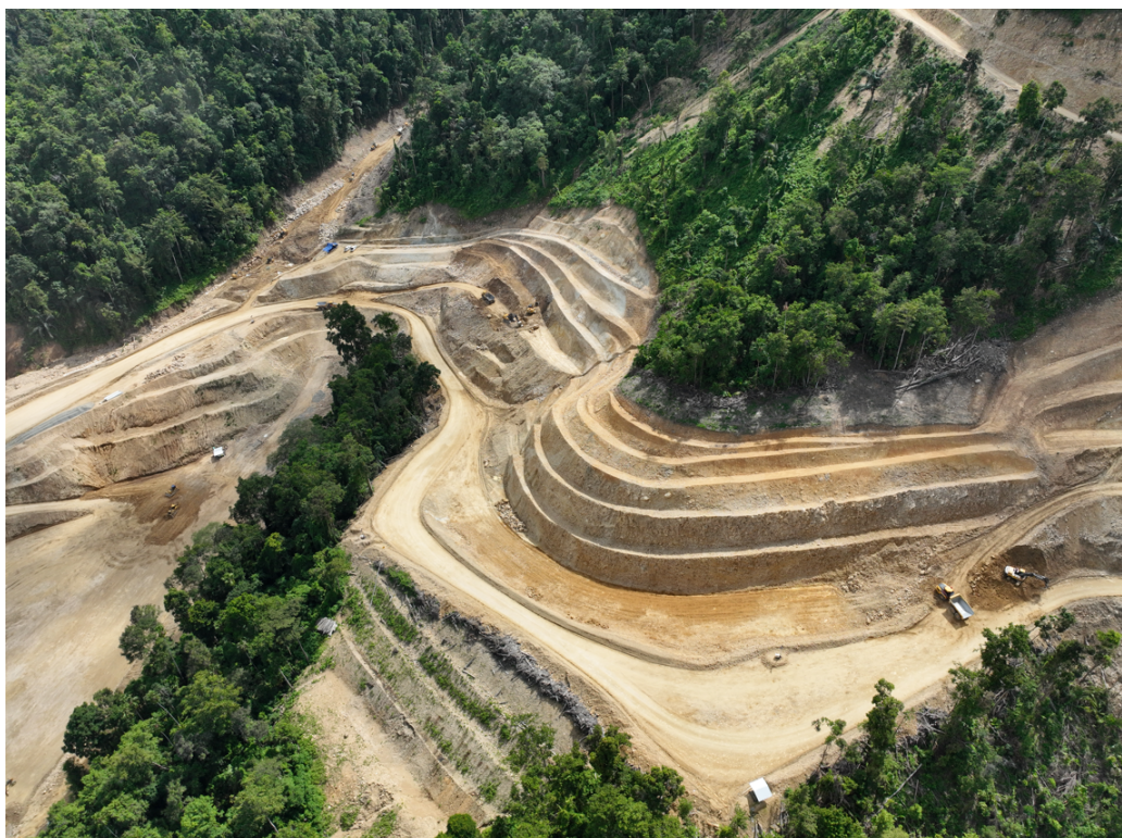
Figure 3: Ore processing plant and mine hauling road construction
