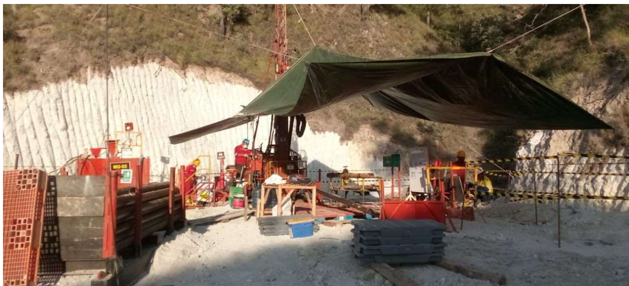
Figure 3: Diamond drilling in regional exploration programs
