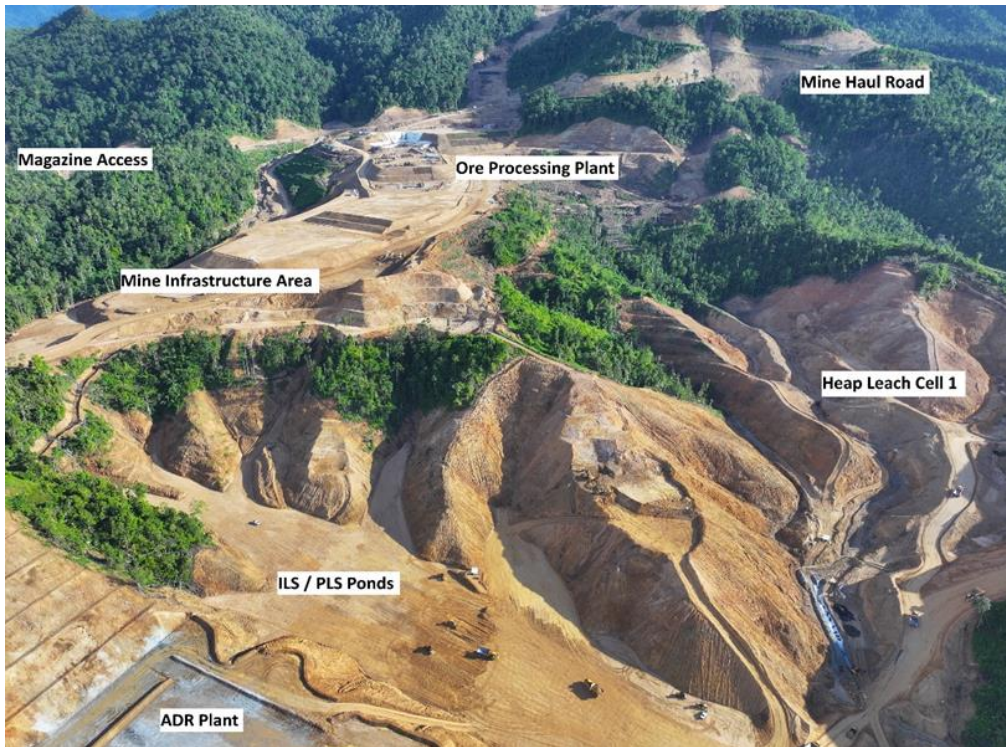
Figure 2: Ore processing plant construction
