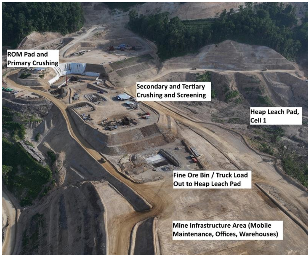
Figure 3: Ore processing plant construction
