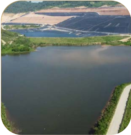
BSI's dam 4 to collect rainwater from heapleach area
