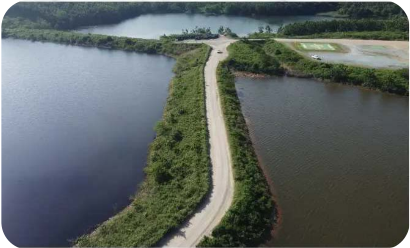
BSI's dam 1, 2 and 3 as environmental control dams
